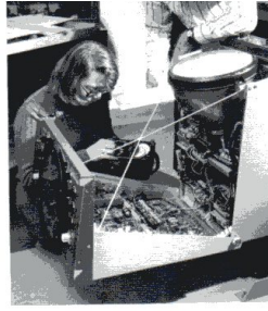
Above. Students checking the circuitry of the Radiolocator 12 radar installed in the radar cabin
